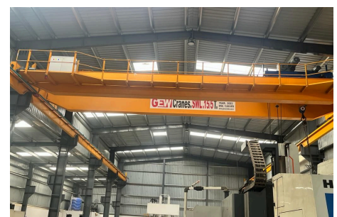
15/5 t double girder crane, workshop installation
