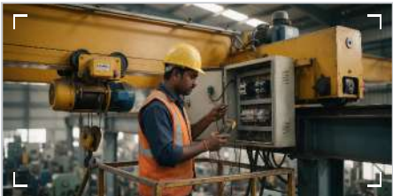
09 Repair & Modernization Mechanical, electrical and safety-system retrofits that extend the life of existing cranes.
